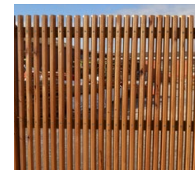
Vertical timber batten screen to substation and drying area
